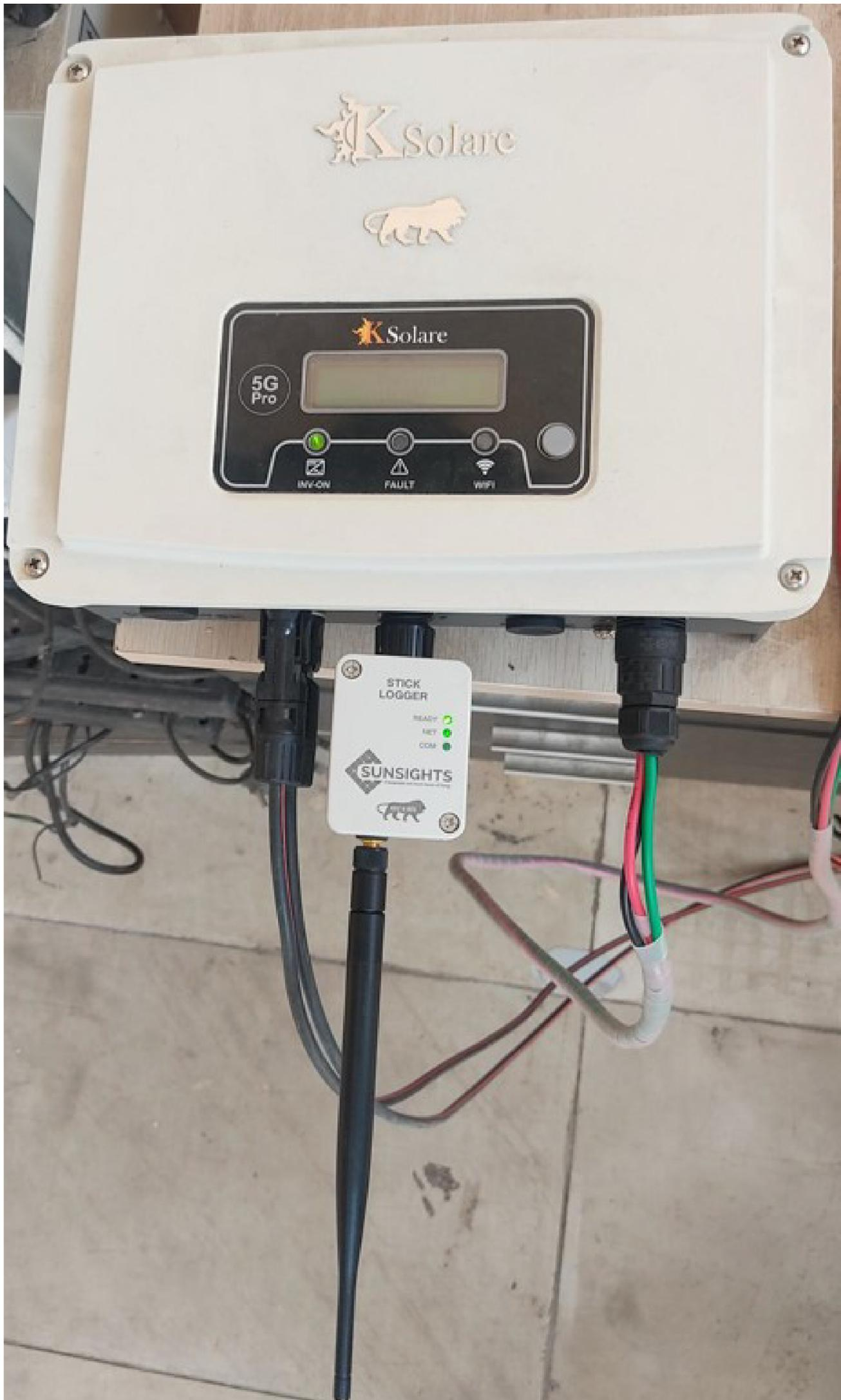
**SunSights RS485 Wi-Fi Dongle [Circular] with KSolare String Inverter.**
