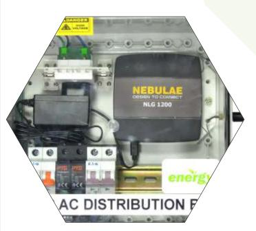
Solar AC distribution box is a central power management box. It connects MCCB, MCB, SPD, Sockets, NebuLink Gateway, etc. This Solar Junction box is fabricated using the latest technology and suitable for different solar power applications. There are various types of distribution boxes, single and three phase, based on the system capacity.
