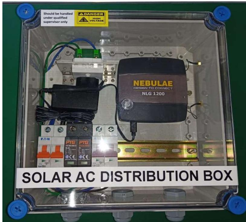
Diagram 6-1: Top View of ACDB (With Enclosure)
